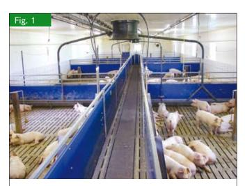
Experimental housing with adiabatic cooling system (water pipes and high-pressure nozzles installed directly in the stable above the windows)
