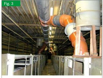
Study design with simultaneous above- and under-floor suction. Air is withdrawn both beneath and above the floor (at a set distance from the ceiling)
